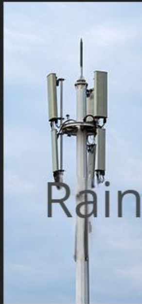
▲ Base station repair and maintenance
