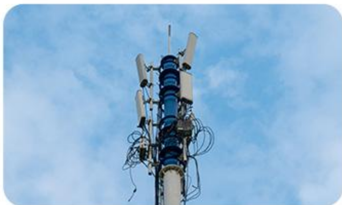
Community installation and maintenance
