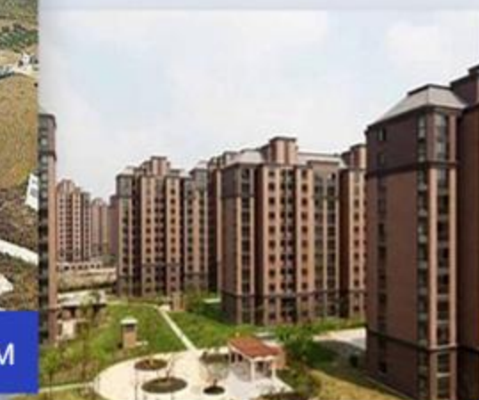
OPTICAL FIBER ACCESS
