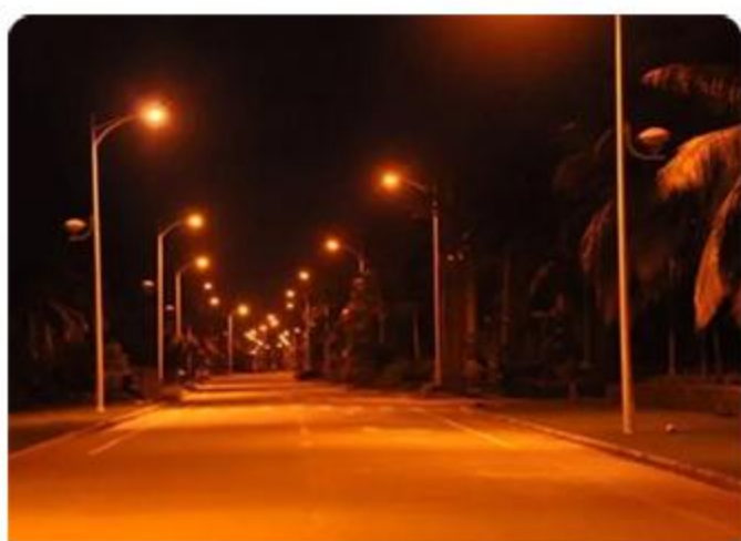
Street light cable maintenance
