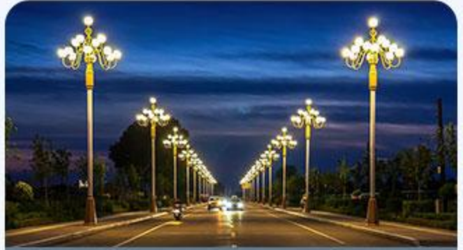
STREET LAMP CABLE MAINTENANCE
