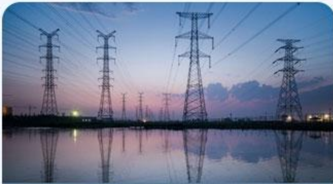
TROUBLESHOOTING OF CABLE FAULT OF RAILWAY COMMUNICATION BASE STATION
